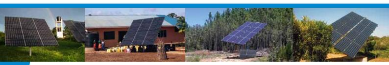
LORENTZ ETATRACK active tracking systems provide up to a 40 % higher yield from your PV modules. ETATRACK systems follow the sun through the day, this extends the time that useful power levels are delivered and maximises the peak power.
